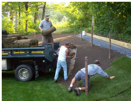
Rising Sun Maintenance crew sodding the hillside for the Incline Railroad installation
